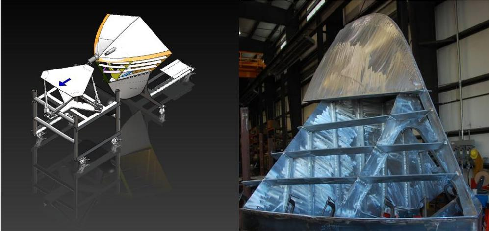
Figure 3, Unmanned connection concept (left) and bow mock up under construction (right)
